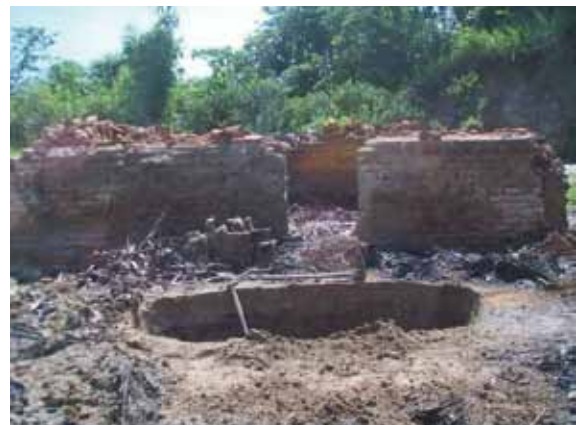
When these brick ovens were destroyed in the 2009 earthquake, 25 Christian families were left without their source of income but Barnabas has now enabled them to build new ovens
