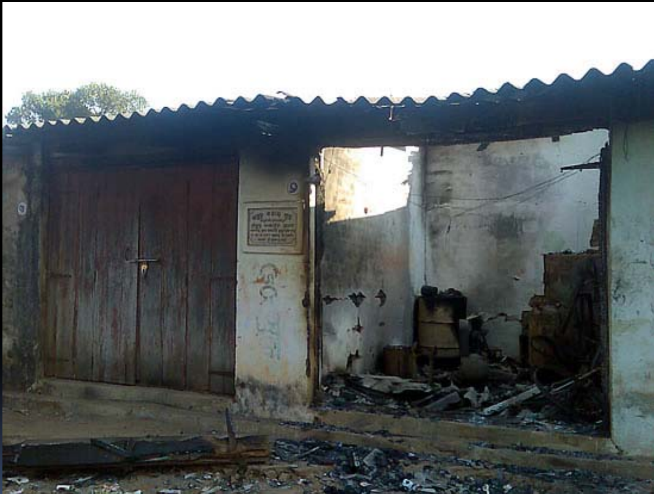
Burnt out shop owned by a Christian
