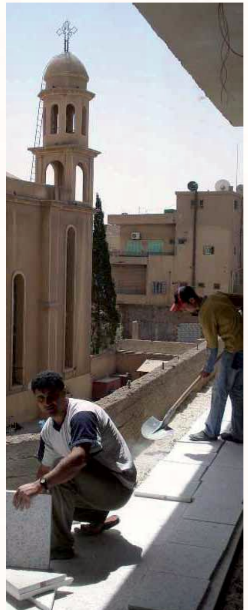
Builders finish work on a new community center, funded by Barnabas
