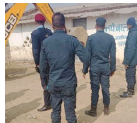
Police oversee the demolition of the church building in Nepalgunj, Nepal
