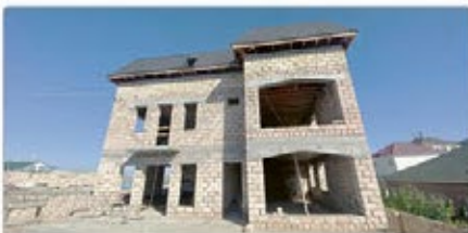
The multifunctional church building takes shape
