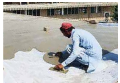
A workman resurfaces a section of the damaged hospital roof
