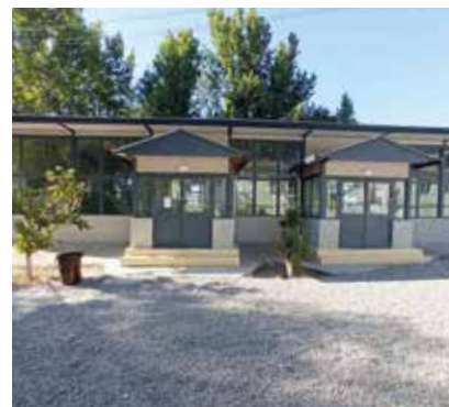
Church volunteers carried out much of the hall renovation themselves
