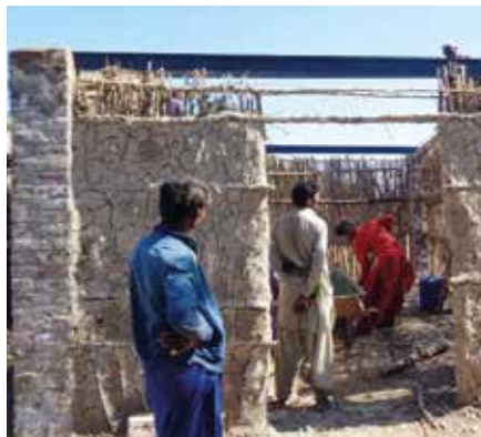
One of the new Barnabas-funded homes under construction, showing the brick-built pillars supporting the mud walls. Some of the iron girders that will support the mud roof are in place
