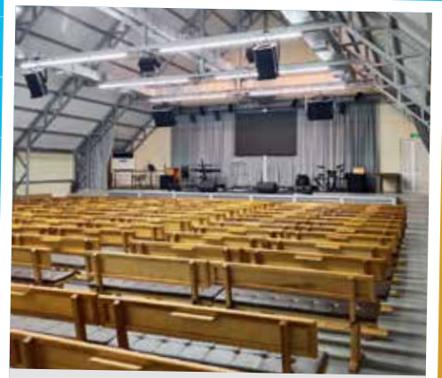
This new Uzbek church building, partially funded by Barnabas, is designed to be easy to dismantle and rebuild.
