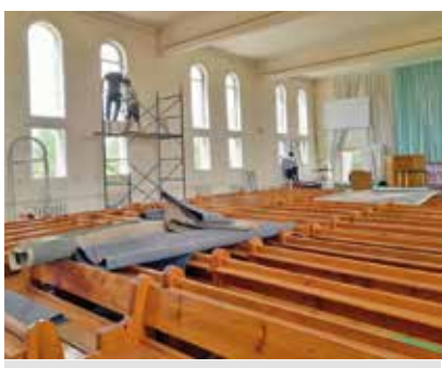
New windows help to keep out the bitter cold
