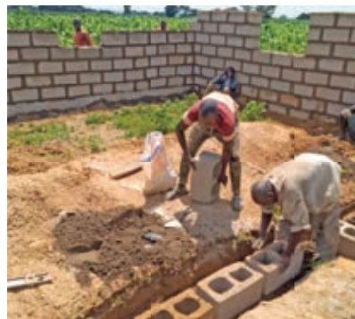
Construction underway on the first two Barnabas-funded health centres
