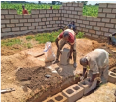
Construction underway on the first two Barnabas-funded health centers.
