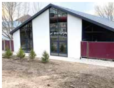
The newly repaired church in Kazakhstan
