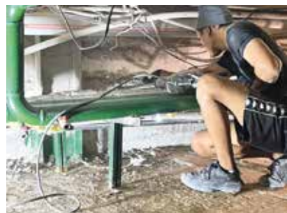
Barnabas-funded work underway on the church basement
